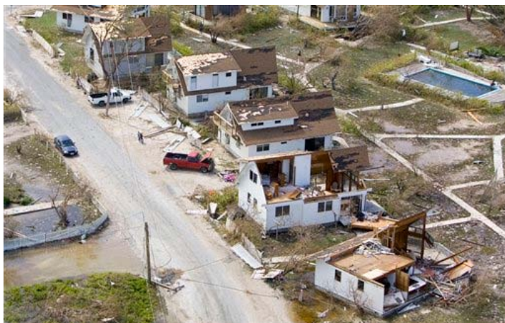
Figure 9: Hurricane Ike damages in Grand Turk
