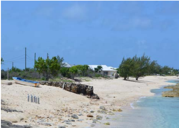
Figure 1: Erosion at Cedar Grove Beach, TCI
